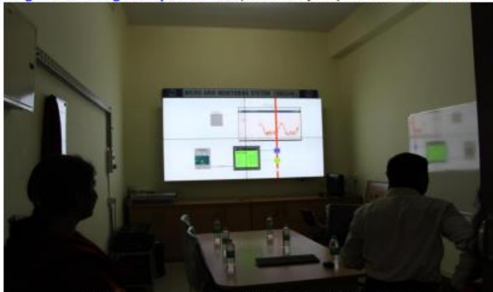
Fig.11. Development of Micro-grid Monitoring Facility @ ICER-IISc
