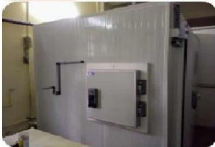
Fig.12 Establishment of Standalone PV thermal system (7ft x 7ft x 7ft chamber) with Desalination system
