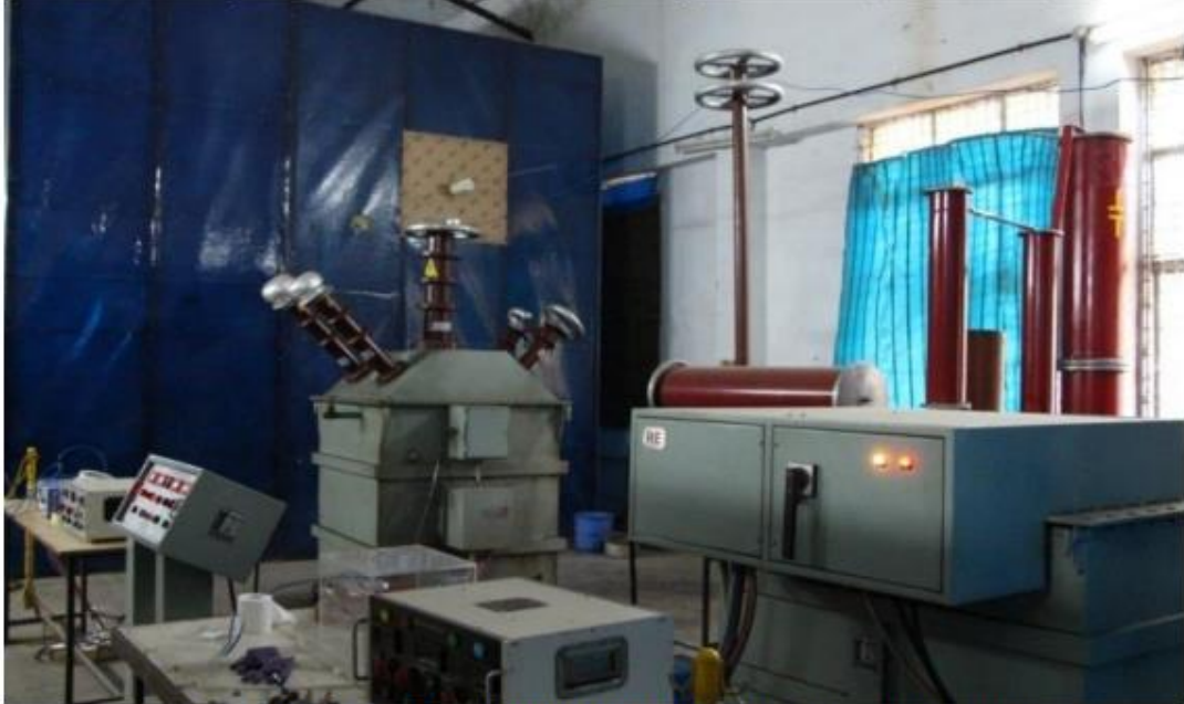
Fig. 1. 150kV AC-300kVA, 250kV/100mA HVDC Artificial pollution facility
